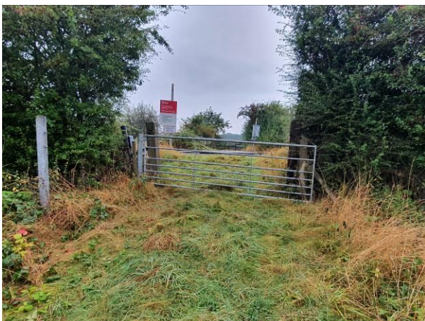
Existing gate to railway line
